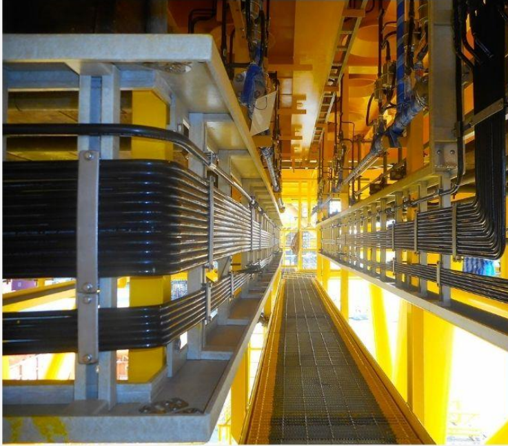
Instrument work Tubing installation
